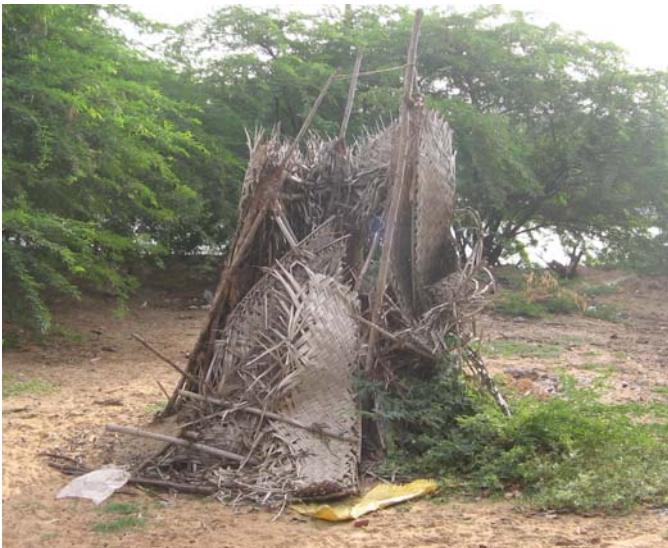
Individual house toilet made from coconut palms.
